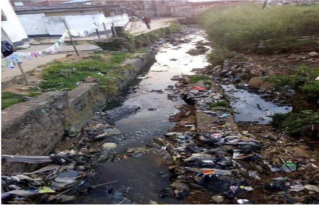
Figure 4.4.A damaged drainage passageway around Yemetu area of Ibadan North LGA with residential buildings around
