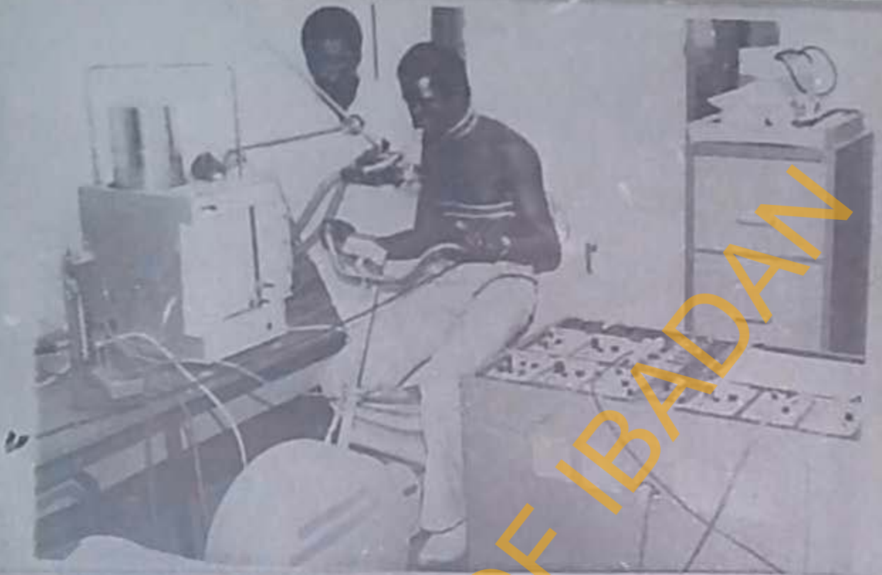
Using the Godhart expirograph, the pulmonary functions of the subject were being determined, pre-exercise.
