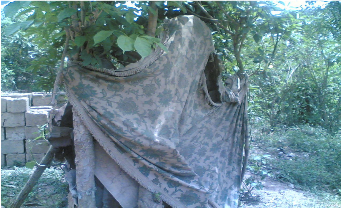
Plate 3.5: A poor bathroom facility in the rural
