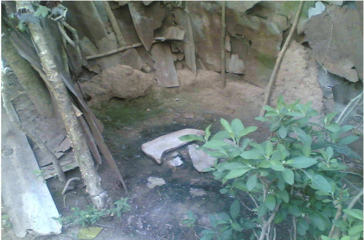
Plate 3.9: Poor pit toilet facility in a house
